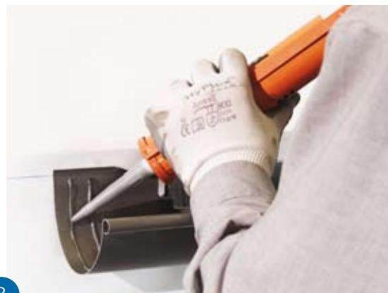
8 Apply 2, thin, parallel lines of adhesive to the inner part of the running outlet.
