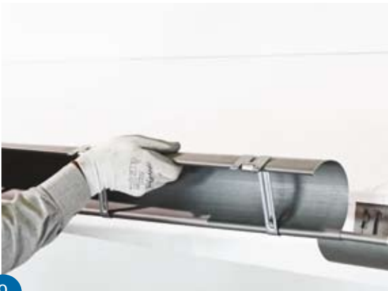
9 Insert the prepared gutter into the already installed running outlet. The adhesive (applied in the previous step) will spread sealing the joint.
