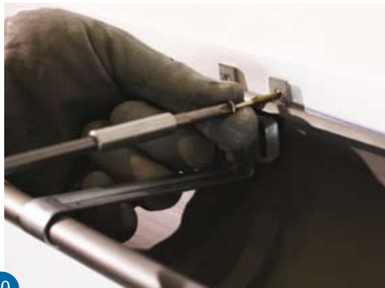
10 Fix the gutter brackets according to the chalkline. Then fit the gutters by their bead first. Ensure 50 mm as min. overlapping.
