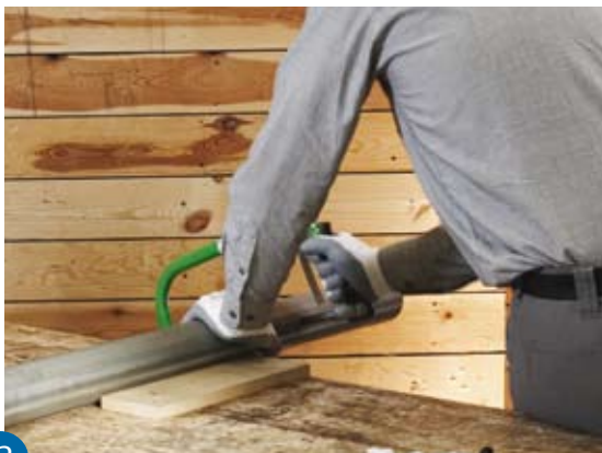
12 Any gutter that requires cutting should be marked using short off-cut. Begin to saw from the beaded edge.
